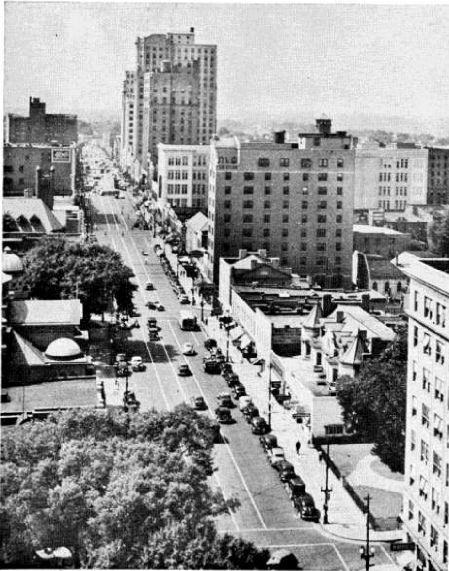
Looking South on North Tryon Street
