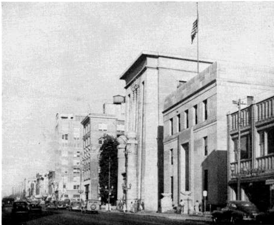
Showing the Federal Reserve Bank and the Masonic Temple, South Tryon Street
